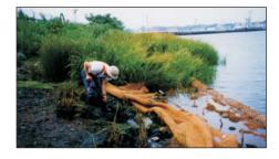
Mason & Associates designed and built a *Spartina alterniflora* saltmarsh at an oil terminal tank farm and site of a former toluene release. The marsh is designed to restore former wetland functions and to reduce residual toxic chemicals through phytoremediation. Mason & Associates has continued to monitor the progress of the restoration in terms of vegetation density and species diversity.
